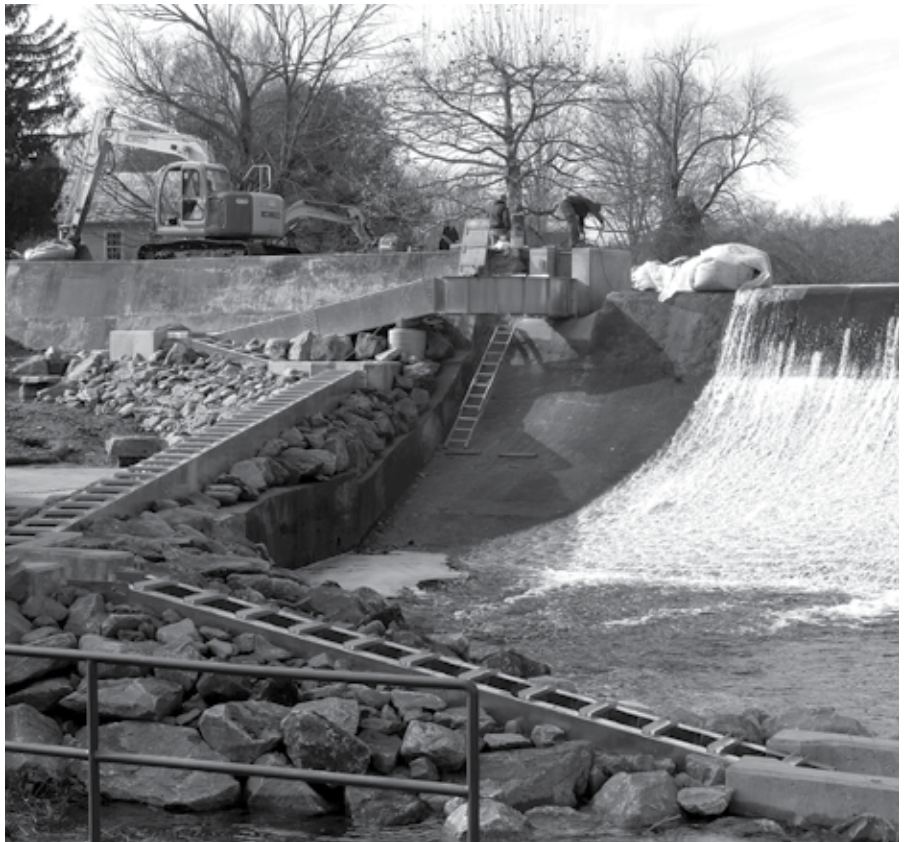
Fishway installation at Centerbrook Architects dam.
