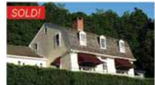
ESSEX • PRISTINE 1790 CENTER CHIMNEY GAMBREL!
